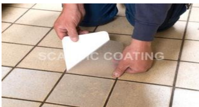
H3405T Clear aqua safe 140mm 140mm being applied A JPG file, 412 KB
